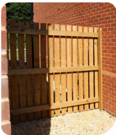
1.8m high close boarded fence between plots D002
